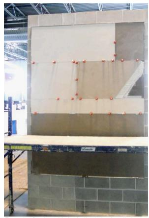
Example of various thin-body tiles being installed using a mechanical edge-leveling system on a vertical surface
