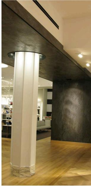
Example of a thin-body, 4.5-mm (4,5 mm) porcelain tile installation on both an interior wall and ceiling header
