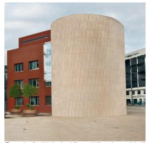
Example of a thin-body, 4.7-mm (4,7 mm) porcelain tile installation on an exterior facade
