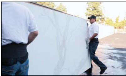
Figure 1: example of light weight Stonepeak large porcelain panel utilizing suction cup handles (see recommended tool guide)
