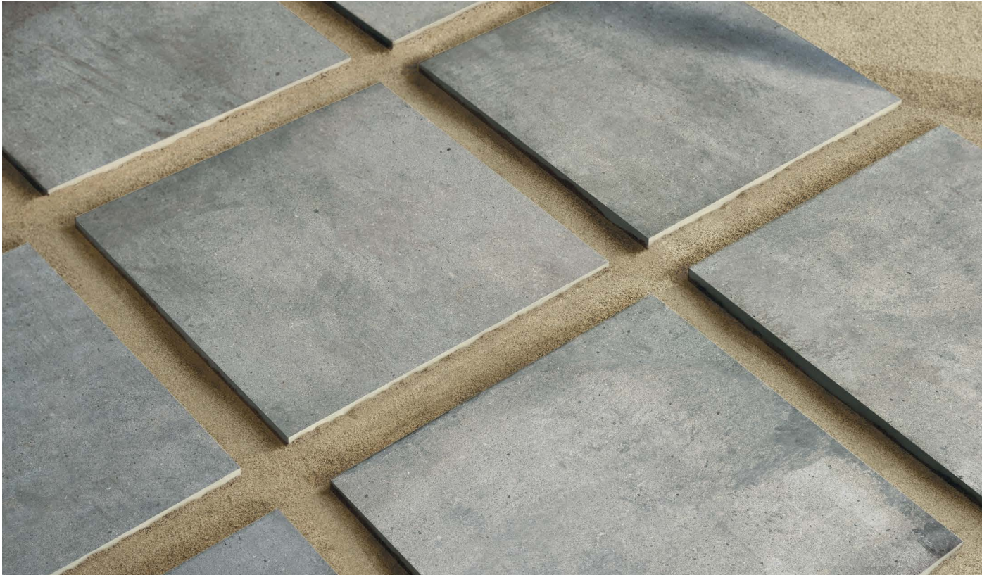
Examples of the dry installation on the sand.
